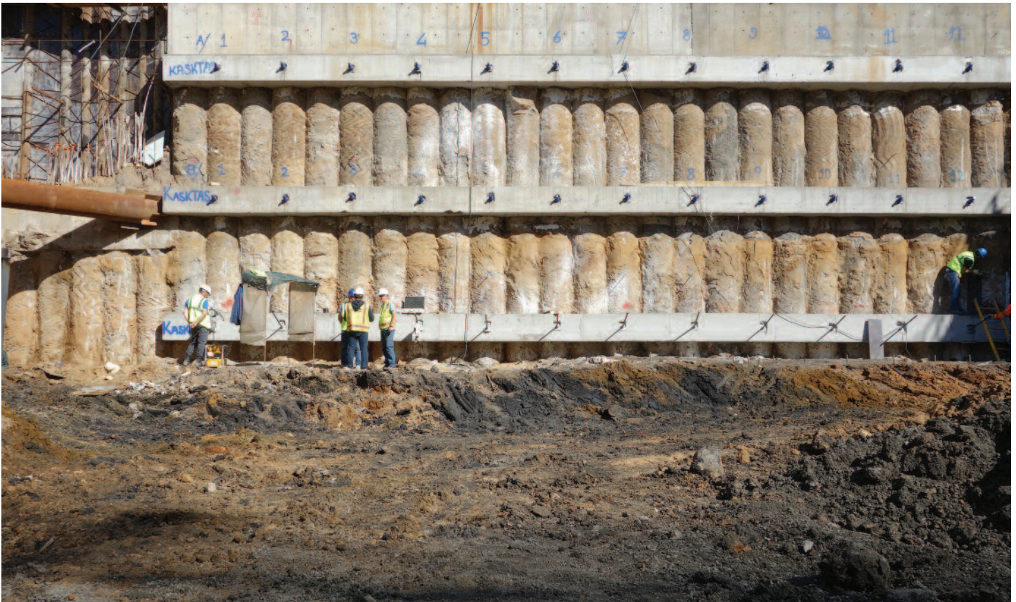
Figure 8 Completed anchored secant pile wall.
